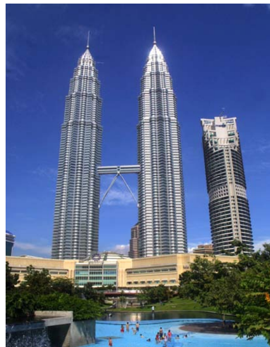
Petronas Twin Towers
